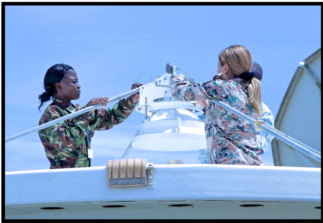
FIGURE 10: MAINTAINANCE of UNOE COMMUNICATIONS EQUIPMENT
