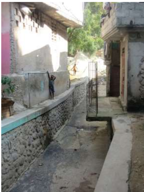
Embankments strengthened at Grann Sonnet
